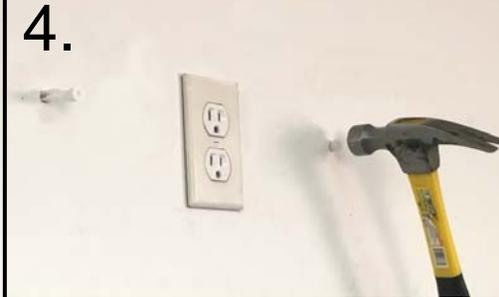
Insert the two plastic keepers that came in the hardware bag into the holes. Using a hammer, lightly tap on the keepers until they are flush with the wall.
