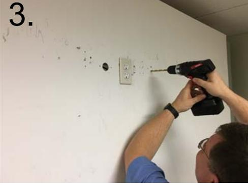
Using the 5/16" drill bit and drill, drill a hole at the two marks on the wall.
