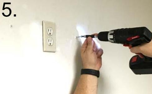
Using a Phillips screwdriver or driver bit and drill, screw in the two screws that were provided in the hardware bag into the plastic keepers. Make sure that you leave the head of the screw approximately 1/4" from the wall.
