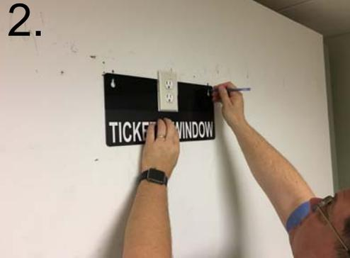
Use the reversible sign to mark the spot on the wall where you are going to install the LED sign with a pen or pencil. Using a tape measure, measure down from the ceiling to the marks you made to make sure that the marks are level.
